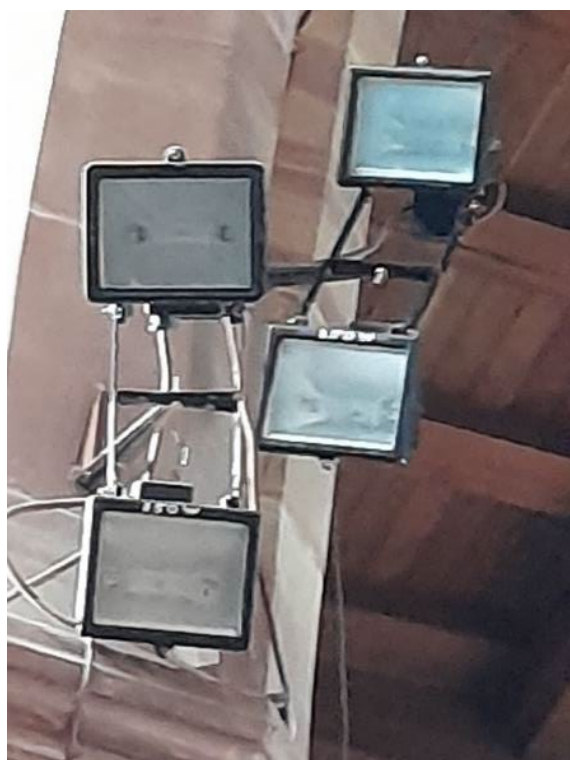
Floodlights using 118mm R7s halogen lamps
