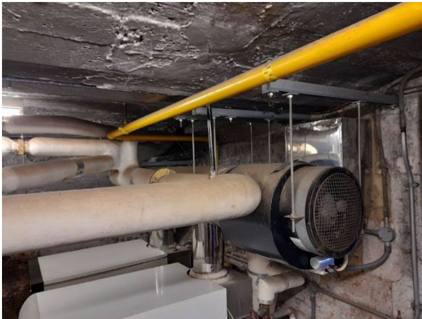
The flue extraction fan, below right.
