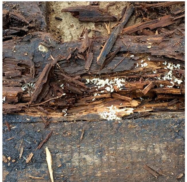
*In areas there was no support at all for the asphalt – which was hanging in mid span. The roof was patched back as far as was possible. However, there is a real danger that as the roof dries out under the patch,*
