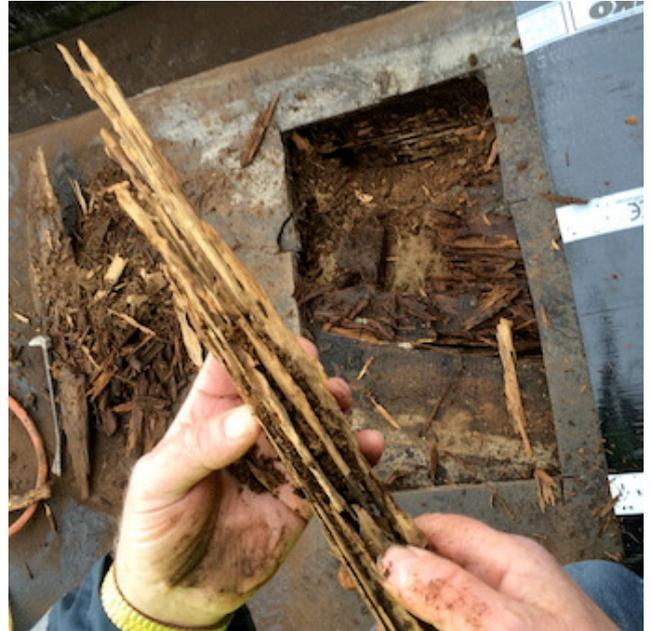
*The boards and edge timbers in this area were wet and one area was found to be heavily infested with larvae.*
